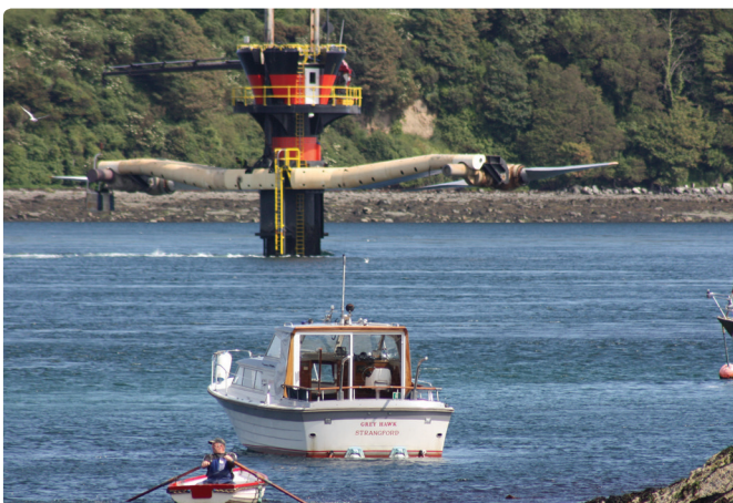
The SeaGen tidal turbine in Northern Ireland with its rotors withdrawn above sea-level (Photo credit: Ardfern, (Own work) CC-BY-SA-3.0 or GFDL, via Wikimedia Commons).
